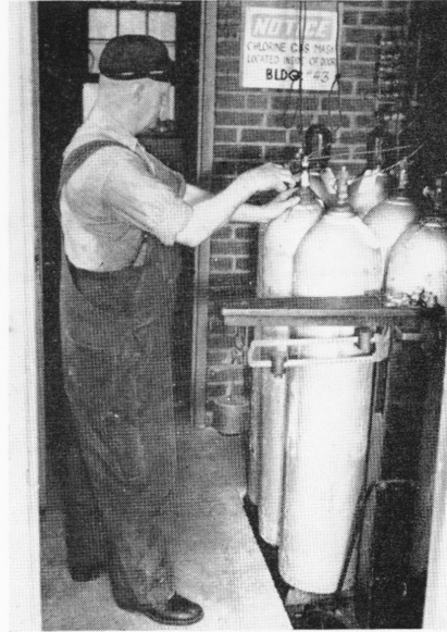
John Theriault, Pipe Shop, daily inspects the four chlorinating stations in the Main Plant. At left above he has just replaced an empty chlorine cylinder with a full one. Note the scale — John can tell exactly how many pounds of chlorine is used in 24 hours. Right, he makes an adjustment on one of the chlorinators located in the West Power House.
